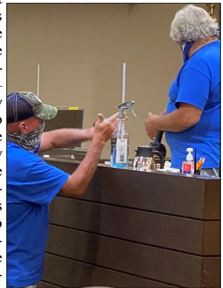
Work crews installing clear plastic shields in a Wilmington courtroom in June 2020.
